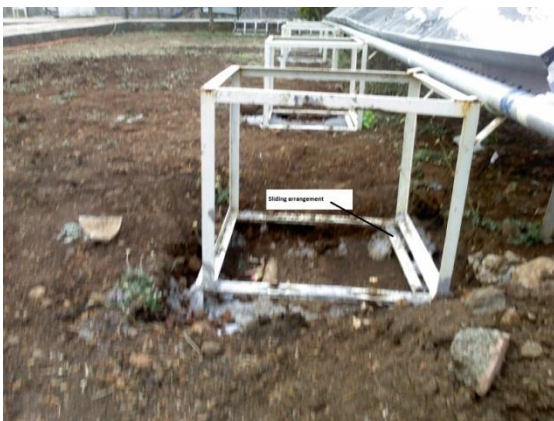
Fig 9: Sliding design of support frames
