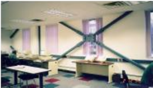
Figure 2 X – braced Friction Damper used in Building
