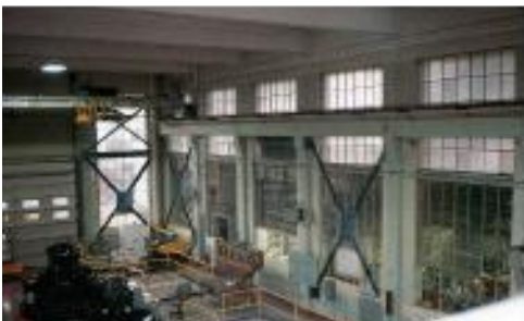
Figure 3 Installation of Friction Damper used in Pump House
