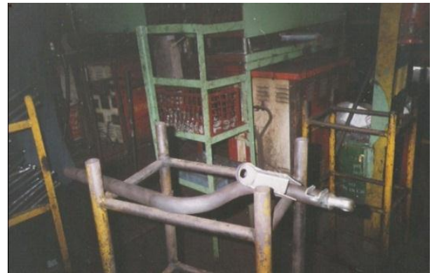
Fig.14 Application of Assembly
