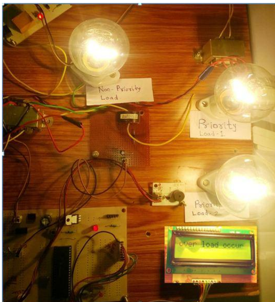
Fig.9. Over load condition of Transformer
