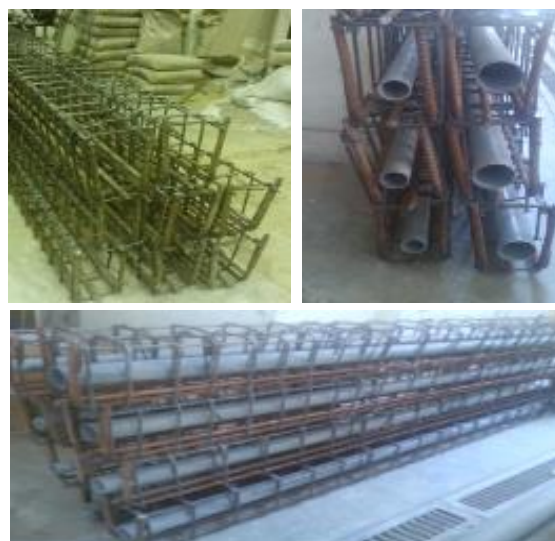
Fig. 4 Reinforcing Cages and Holding PVC Pipes
