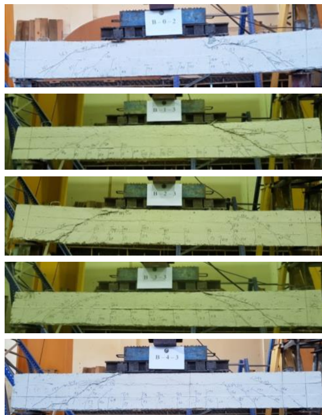
Fig.13 Crack Pattern for Beams with Over Reinforced Section
